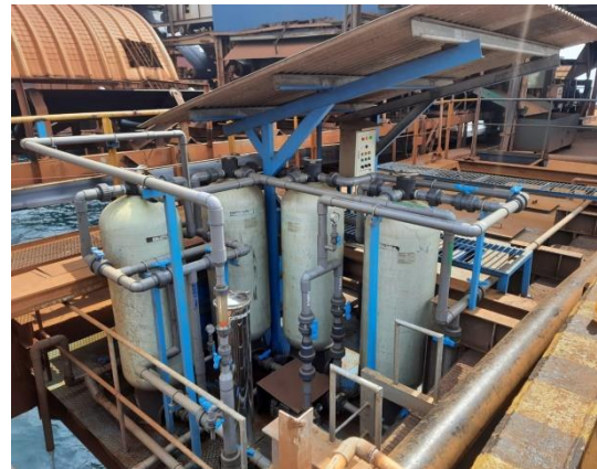
Waste Water Treatment Plant Jetty
